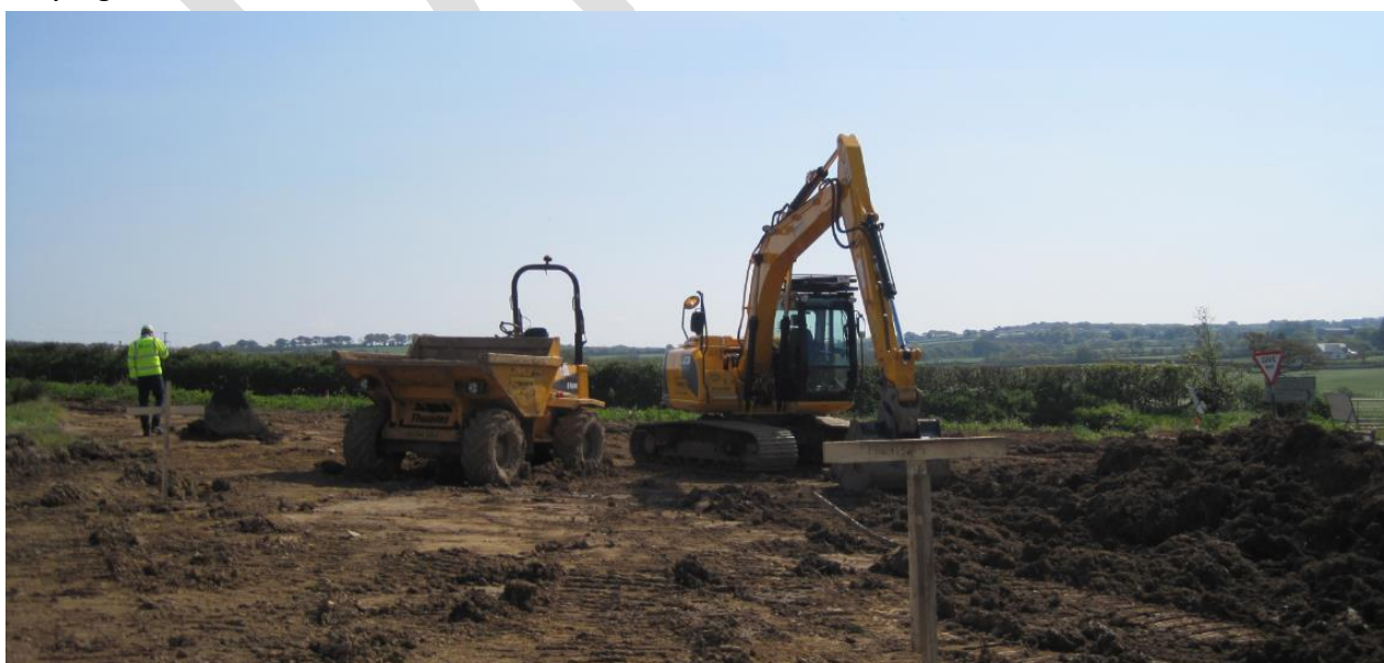
Holsworthy Agri-Business Centre Access 2014
