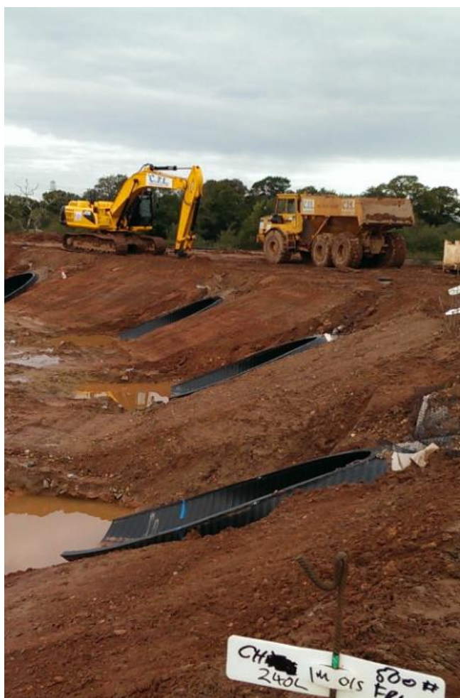
Cranbrook Rail Station access road 2014
