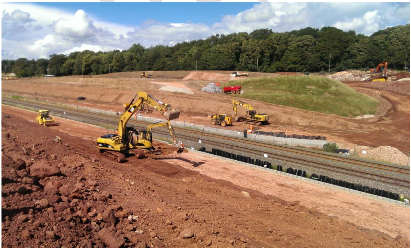
Aller Railway Tunnel 2014
