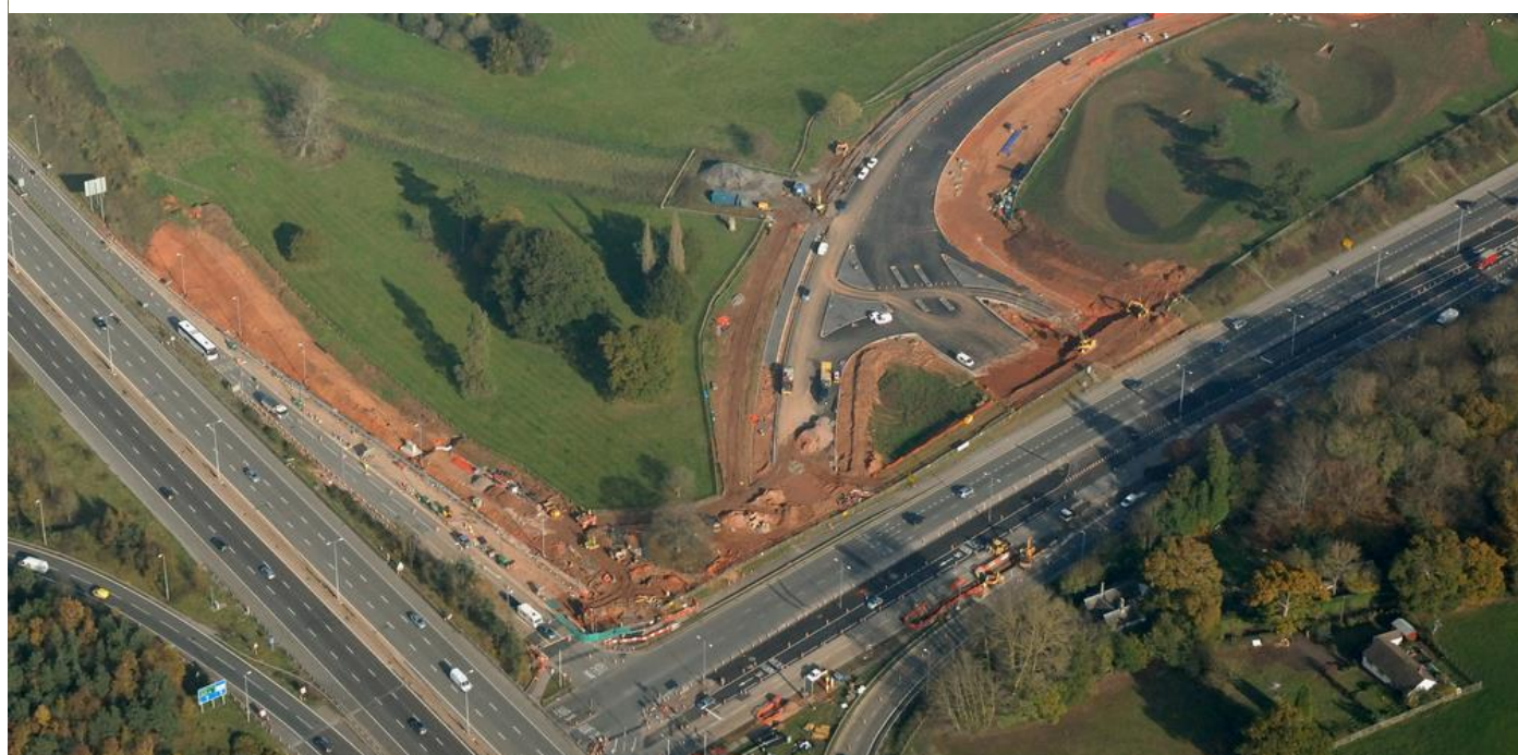
M5 Junction 29 Improvements 2013
