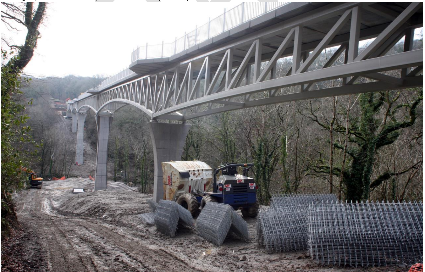
Gem Bridge (near Tavistock) Pedestrian / Cycleway 2013
